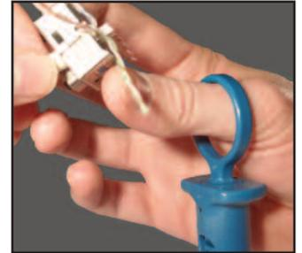
Untwisting wires sounds easy, doesn't it? It might sound easy to anyone who doesn't do a lot of it. The truth is that more time is dedicated to preparing a cable than to actually terminating it, and the longest part of the preparation process is untwisting wires. It is also one of the largest determinates to the ultimate speed, loss, and cross talk. So, proper cable preparation is an absolute necessity in order to obtain the desired performance.
