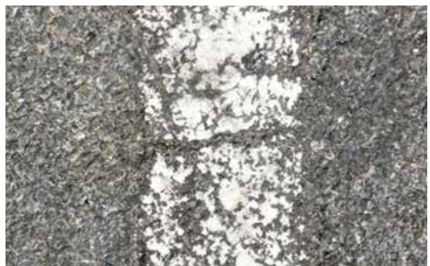
Barely visible marking. Worn road markings lead to a poor luminance level.
