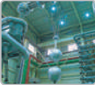
High Voltage Test / Impulse Test
