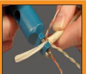
Easily cuts the cable filler with the cable filler shear.
