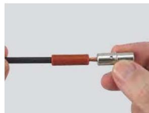
**Step 3:** Insert wire into barrel of contact and crimp using designated tooling.
