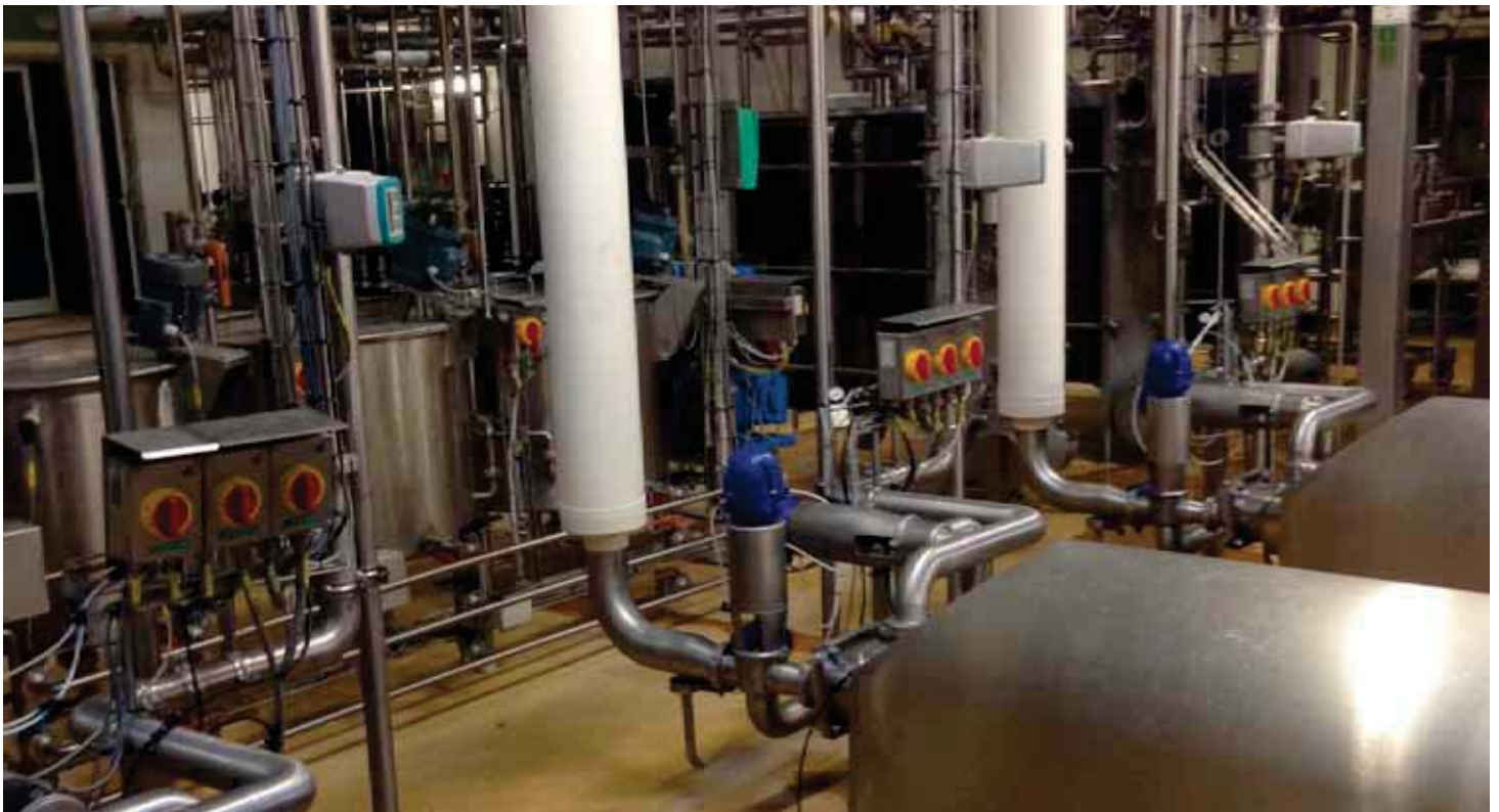
Stainless steel safety switches at Arla Foods
